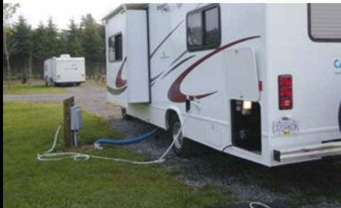
1011.2.1 Clear Ground Space Utility and sewage hookups
